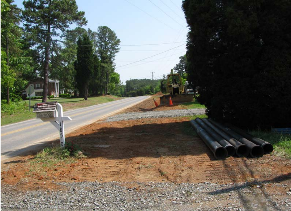
Waterline construction east on Virginia Road
