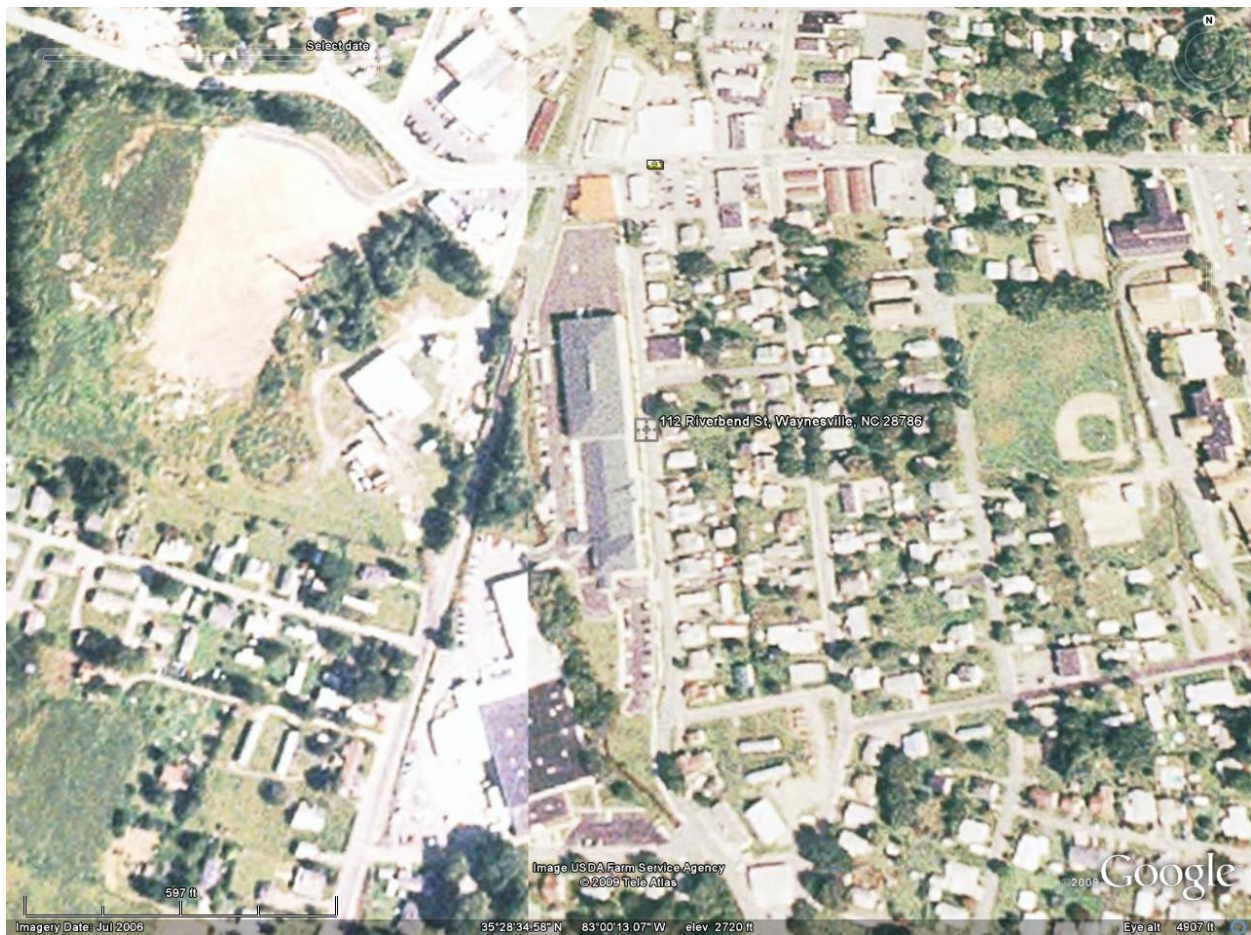
Figure 4. 2009 satellite view of the Benfield Industries NPL site showing the Hazelwood Vocational Opportunities facility re-development of the site (Google Earth).
