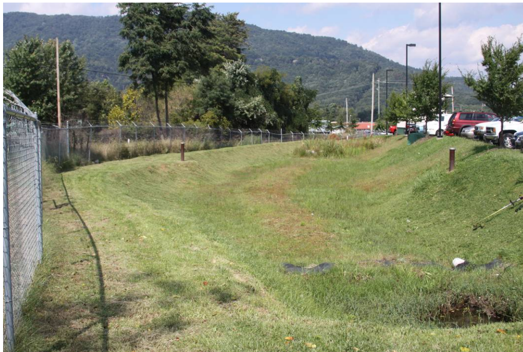
Figure 9. Benfield Industries NPL site, September 2009. View facing north-northwest inside HVO secured area. View of storm water collection pond, security fence and 2 monitoring wells.
