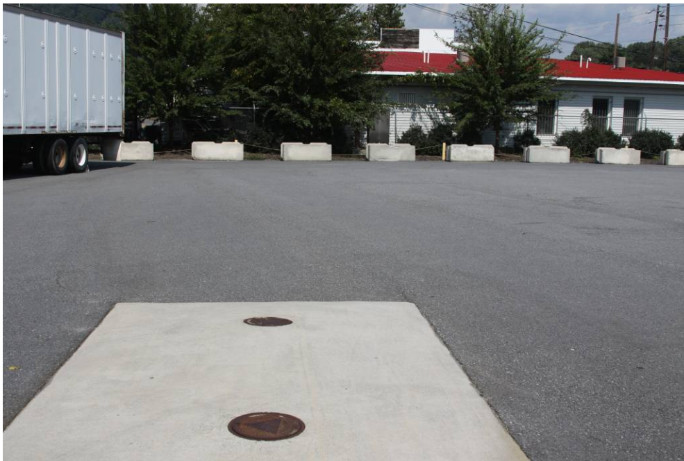
Figure 11. Benfield Industries NPL site, September 2009. North perimeter of Benfield Industries NPL site. View of security fence and commercial building beyond north side of site. Monitoring wells are visible in the foreground.
